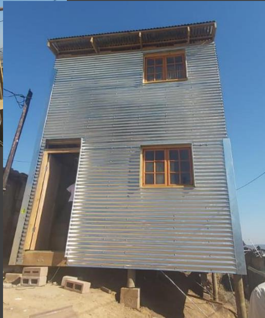
External cladding being installed
