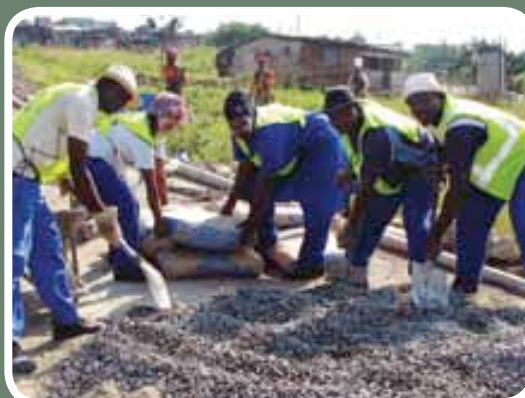
A local construction team mixes the concrete which will be used on the new road being built in Redcliffe informal settlement.
