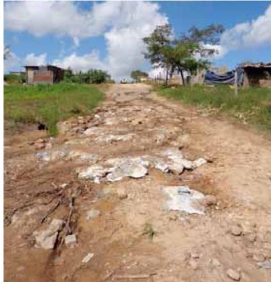
Uncontrolled runoff has eroded secondary roads in the settlement to the point where they are virtually impassable.
