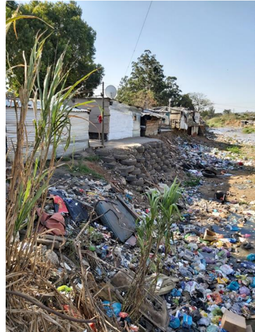
Photo 1: Quarry road: Waste thrown into the river
